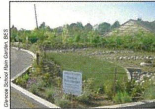
Opportunity for a Rain Garden. At Glencoe, the Rain Garden relieves sewer back-ups by infiltrating stormwater, improves water quality, and provides an aesthetic & education amenity to the school & community
