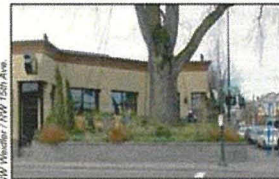
Grade Separation for Outdoor Seating
