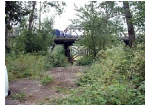
9. Approaching end of alignment at N. Portland Road bridge.
