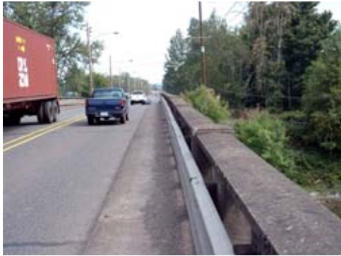
10. Looking north from southern end of N. Portland Road Bridge.
