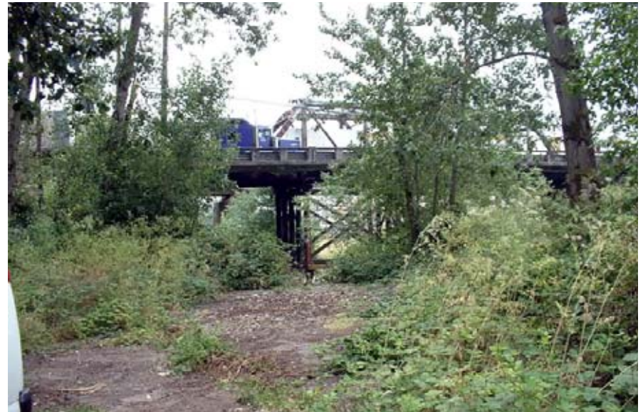
North Portland Road bridge over Columbia Slough
