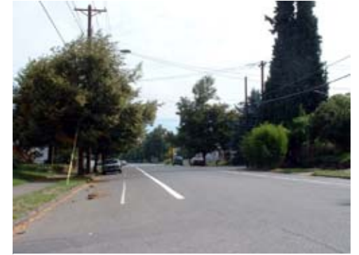
12. Existing bike lanes on N. Smith Street.
