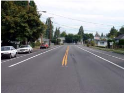
13. Existing bike lanes on N. Fessenden Street.
