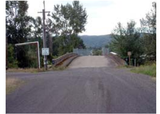
9. Looking south towards Forest Park from north side of landfill bridge.
