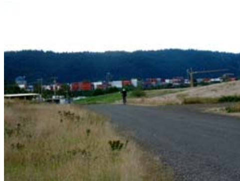
5. Heading west toward landfill entrance on southern perimeter landfill road.
