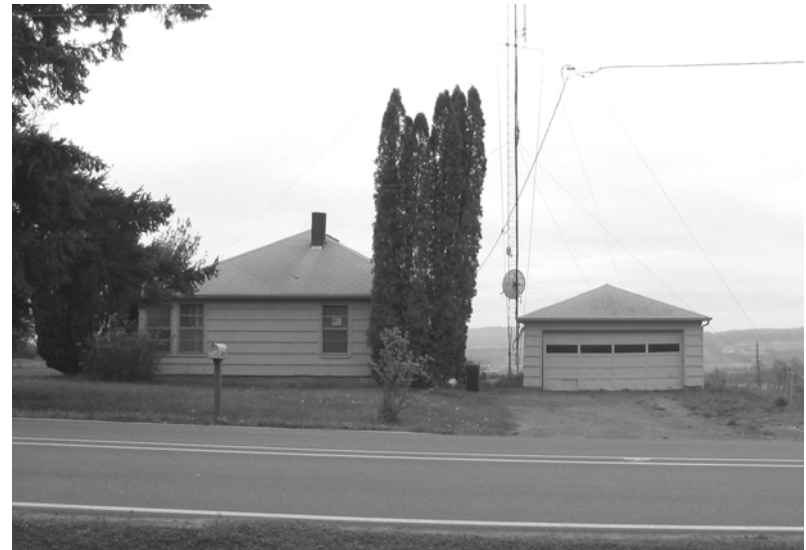
Existing structures along Kemmer Road
