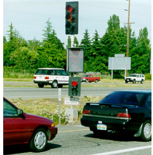
*Ramp metering reduces the delay associated with traffic merging onto freeways.*
