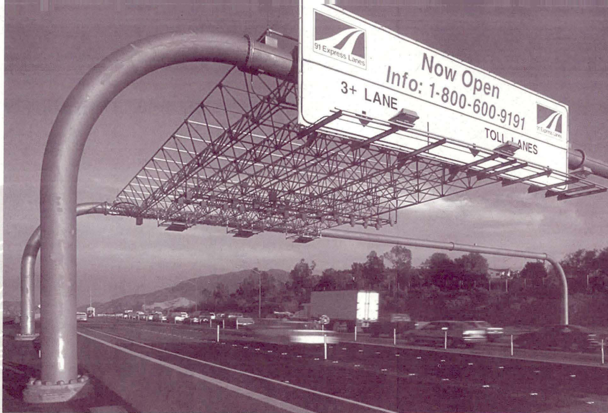
Automatic vehicle identification technology is used on State Route 91 in Southern California.
