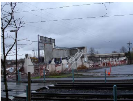
Westgate Theater Demolition
