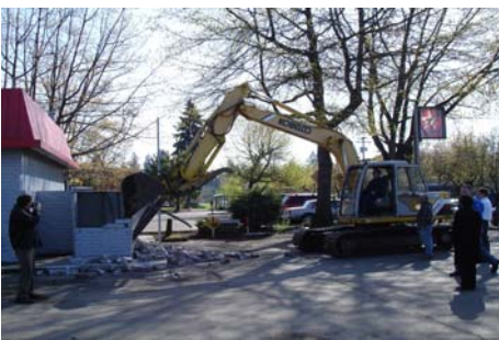
Milwaukie Town Center Demolition
