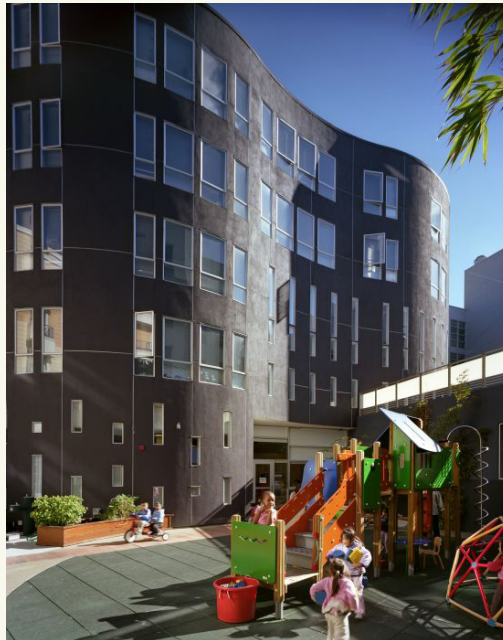
A project by SOMA Studios has unbundled the cost of parking from the sale of units Photograph provided by David Baker + Partners
