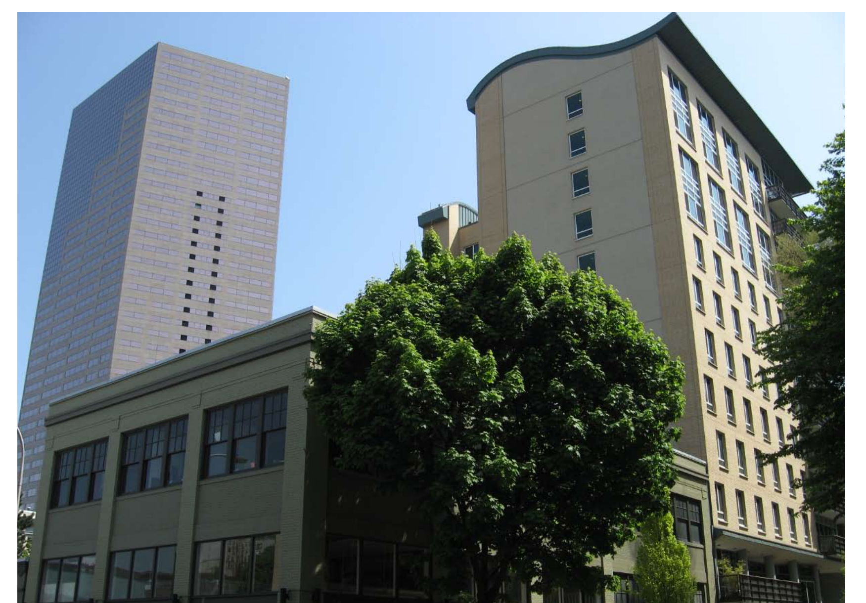
The Central City Concern building, at right above, provides 180 units of transitional, affordable housing in downtown Portland.
