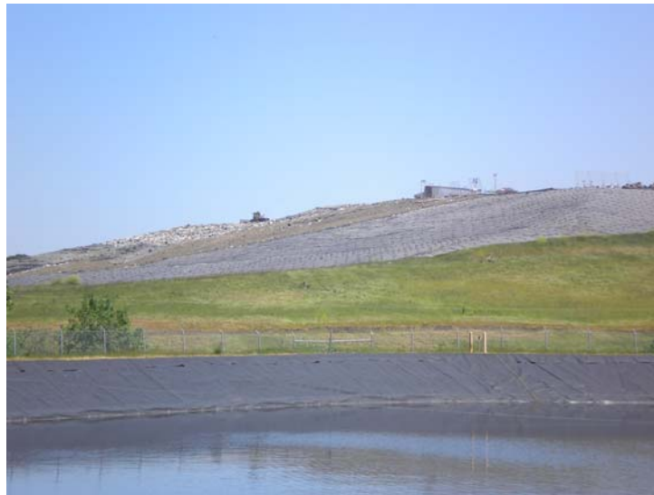
Riverbend Landfill – Leachate retention pond in the foreground; working face of the landfill in the distance
