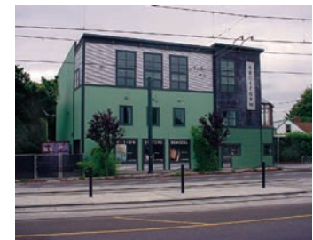
Public investments in corridor amenities like light rail can spur private development as shown in these before (top) and after photographs.
