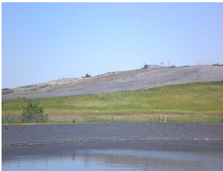
Riverbend Landfill – Leachate retention pond in the foreground; working face of the landfill in the distance
