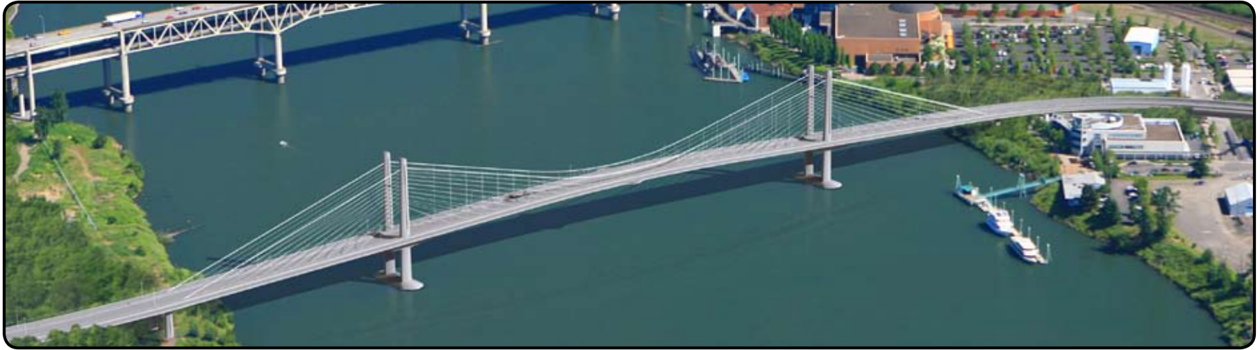
Conceptual rendering of a cable-stayed-suspension hybrid bridge type as viewed from above.
