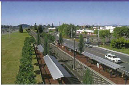
With light rail – Main Street Station
