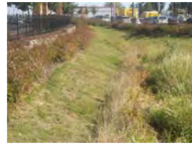
Stormwater swale
