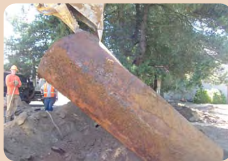
As part of the assessment under this grant, the extensive soil sampling included removal of four underground storage tanks.
