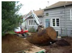
Tank removal on site
