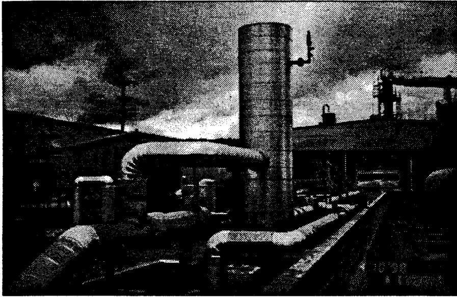
The Ash Grove metering station continuously monitors methane content and flow rate.
