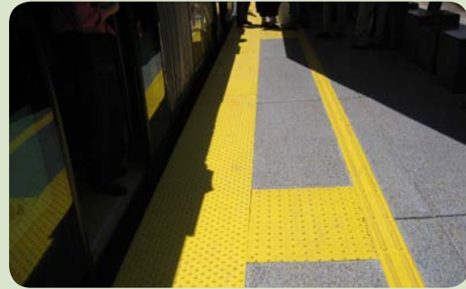
Tactile strips at stations
