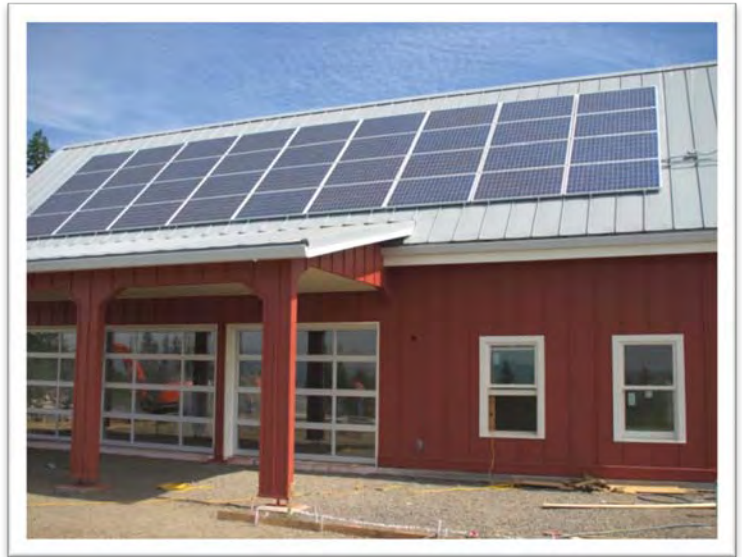
Installation of solar array at Metro's Cooper Mountain Nature Park, 2009.
