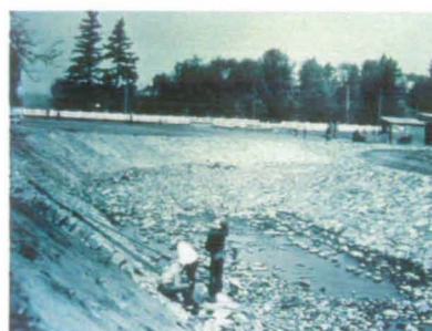
WPA rock lining and channelization (1930s)
