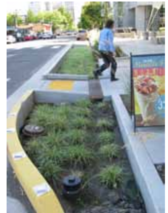
Stormwater drainage doubles as a curb extension.
