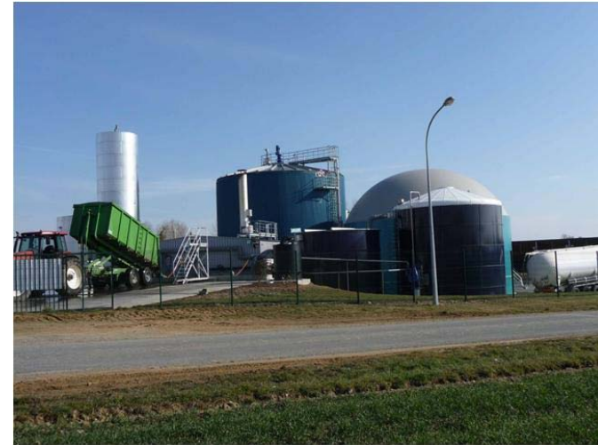
Gicon AD Plant, Biogasy, France
