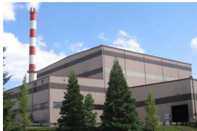
Marion County, OR. WTE Facility
