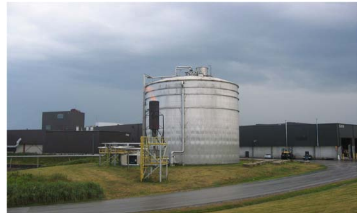
Dufferin AD Plant, Toronto, ON.
