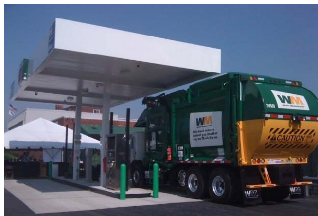
CNG Station, Camden, NJ.
