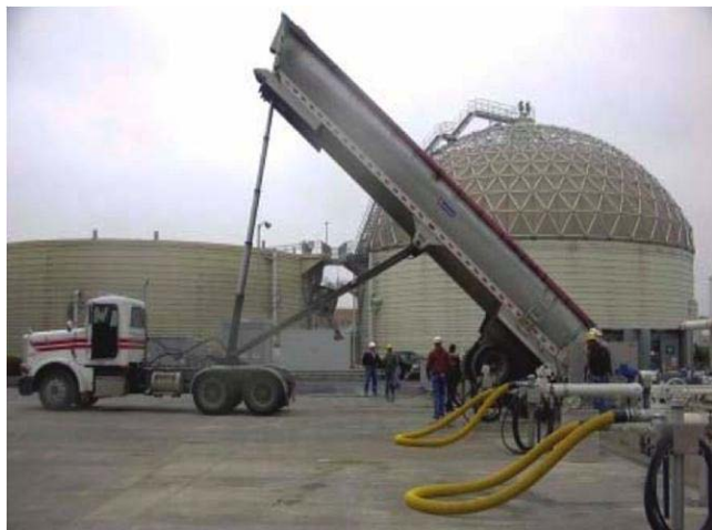
Wet AD, East Bay MUD., CA.
