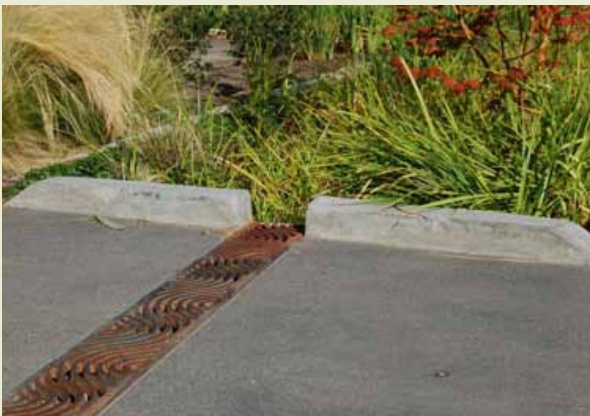
FIGURE 17: EXAMPLE WATER CAPTURE SYSTEM, GRATE AND BIOSWALE
