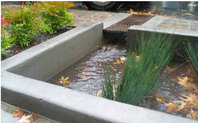
Open space and built amenities, like bioswales that catch stormwater, contribute to water quality and natural systems.
