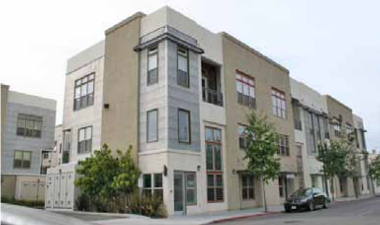
Three-story, mixed-use development in Portland.
