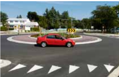
Example of a roundabout
