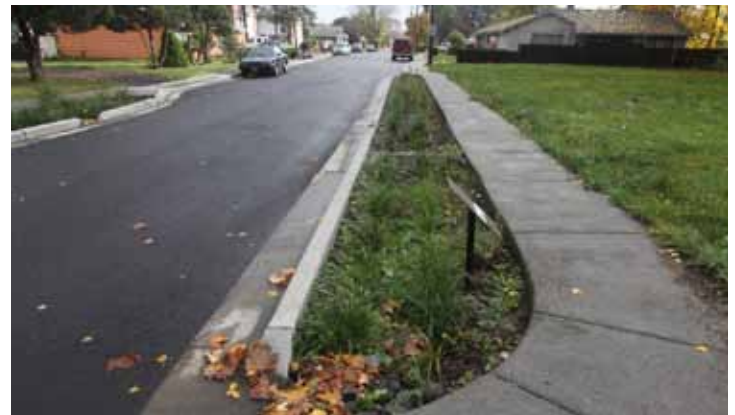
Beaverton's green street treatment on SW 7th Street manages stormwater runoff.
