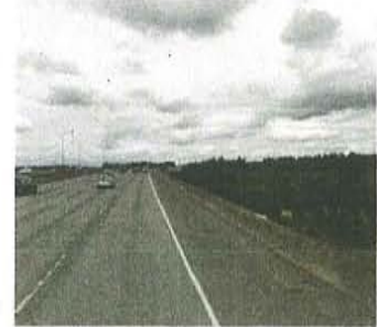
Glenn L. Jackson Memorial Bridge Interstate 205 - Columbia River
