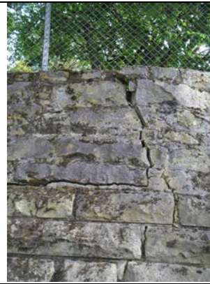
Crack SE Corner of wall
