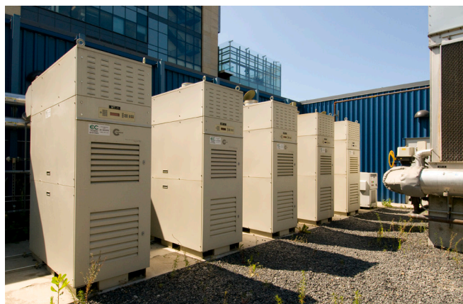
Microturbines at OHSU-South Waterfront
