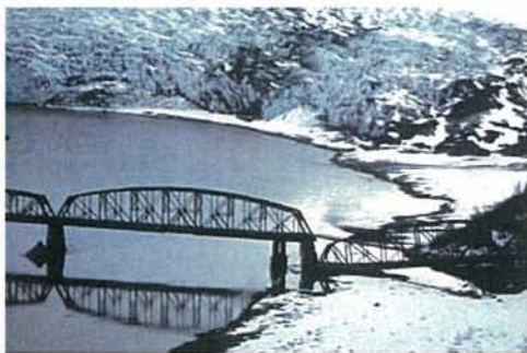
A span of the "Million Dollar Bridge" in Alaska slipped off its foundation during an earthquake in 1964.
