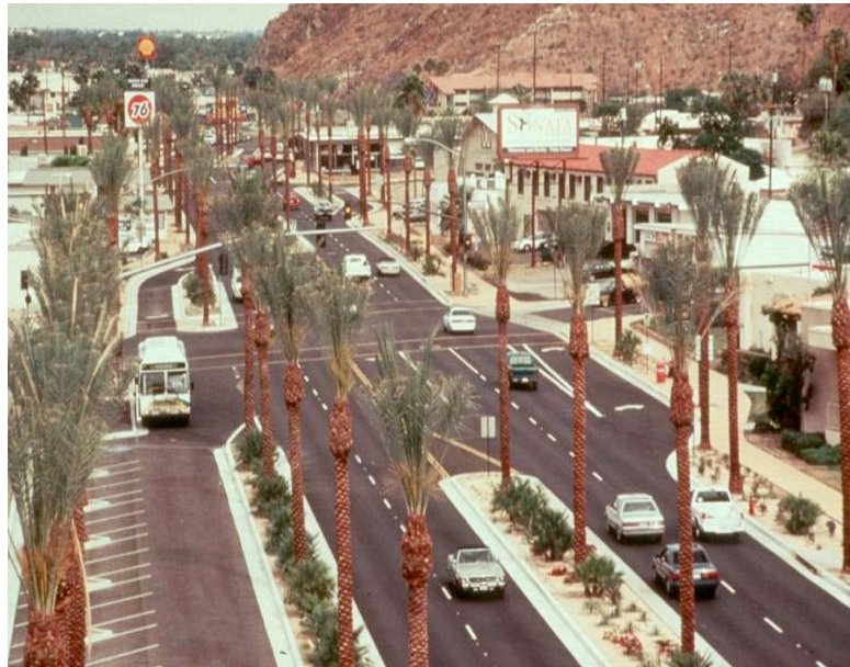
Reconstructed SR 111 with roadway capacity focused at intersections, landscaped boulevard with medians, service drives, for parking and bus stops.
