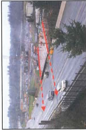
The new bridge, currently under construction on the west side of the highway, will slide into its permanent position.
