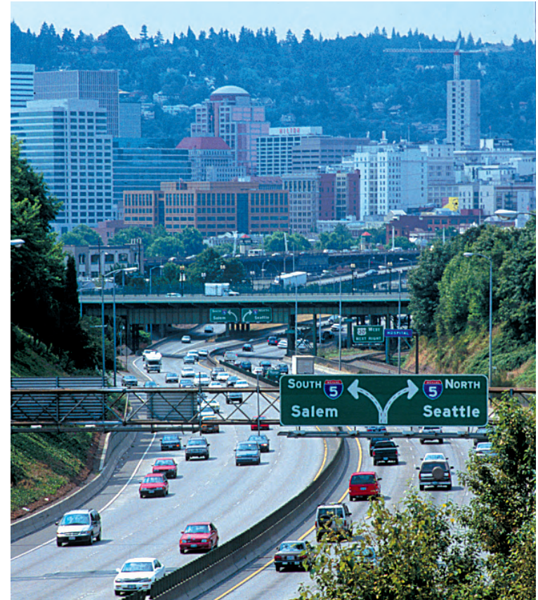
Freeways allow people and goods to connect to major destinations across the region, accommodating longer-distance regional and state-wide travel and providing important access to the region’s major activity centers, such as downtown Portland, and freight access to industrial areas and freight intermodal facilities.
