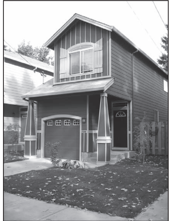
(Two-story townhouse without level entry)
