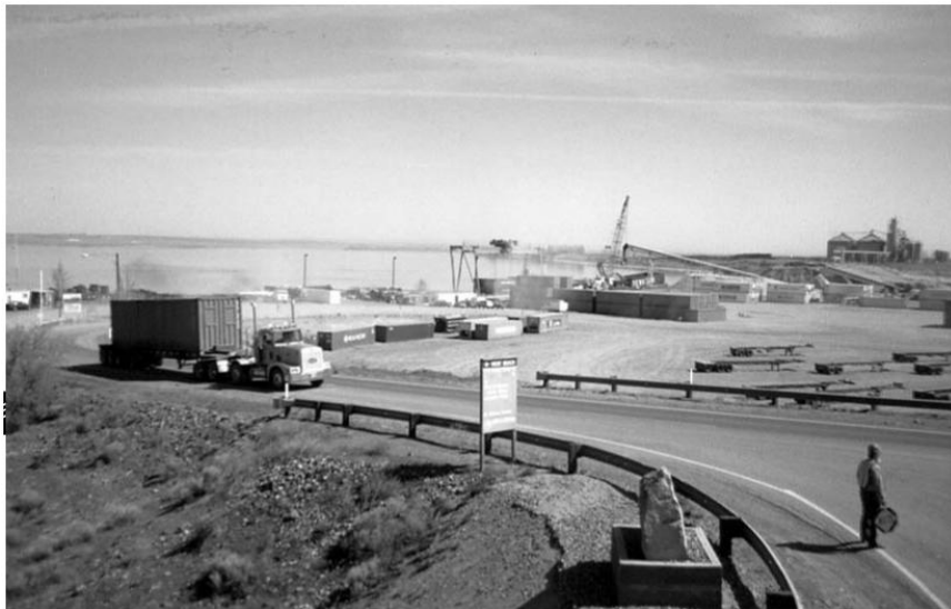
24 The intermodal connector at the Port of Morrow connects Interstate 84 to port facilities where 25 goods are transferred from truck to barge. (Photo courtesy of Port of Morrow) 26
