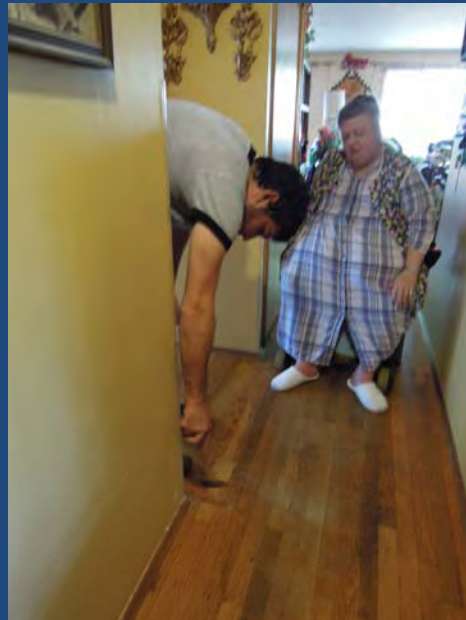
Emergency Adapt-A-Home Safety Repairs
