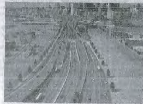
SOUTHERN TUNNEL PORTAL: 13 LANES OF CEMENT
