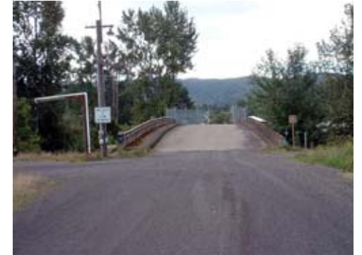
6. Looking south towards Forest Park from north side of landfill bridge.
