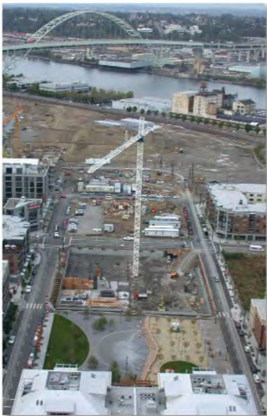
Pearl District, Portland Parks and housing under construction
