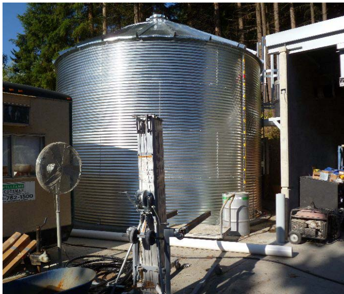
A 30,150 gallon tank captures rainwater from the Oregon Zoo's new Veterinary Medical Center.
