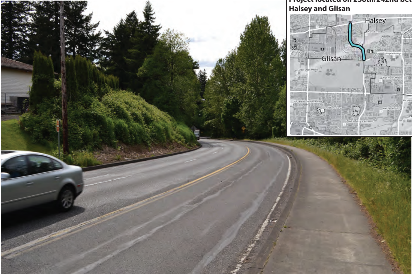
Existing 238th - looking north
