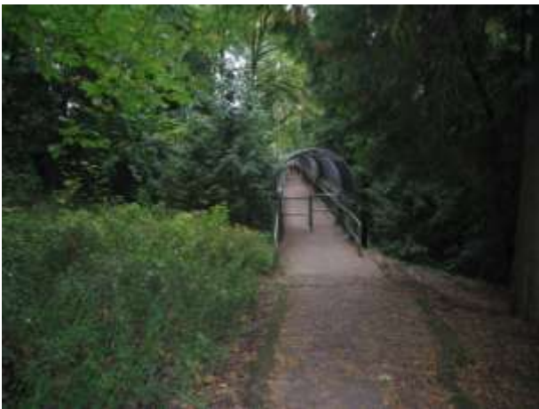
A pedestrian bridge crosses Trillium Creek near Robert Gray Middle School. Photo: The Oregonian
