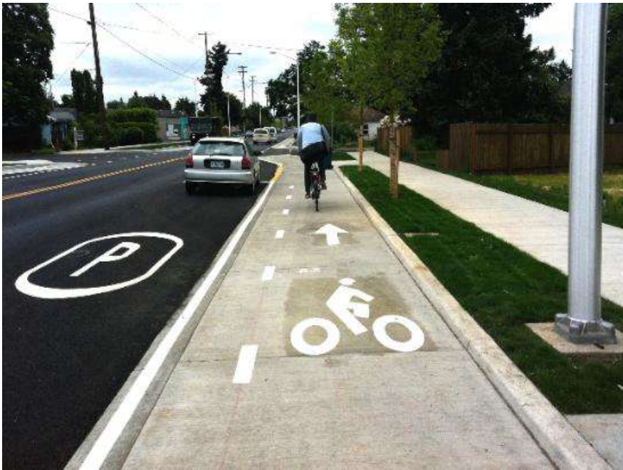
Example of a raised cycle track that is a Bicycle Parkway. Cully neighborhood, Portland. Photo: BTA
