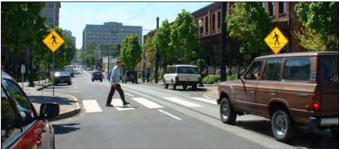
Treatments such as pedestrian crossings improve the viability of pedestrian to cars and trucks. Photo: Federal Highway Administration Pedestrian Safety Plan
