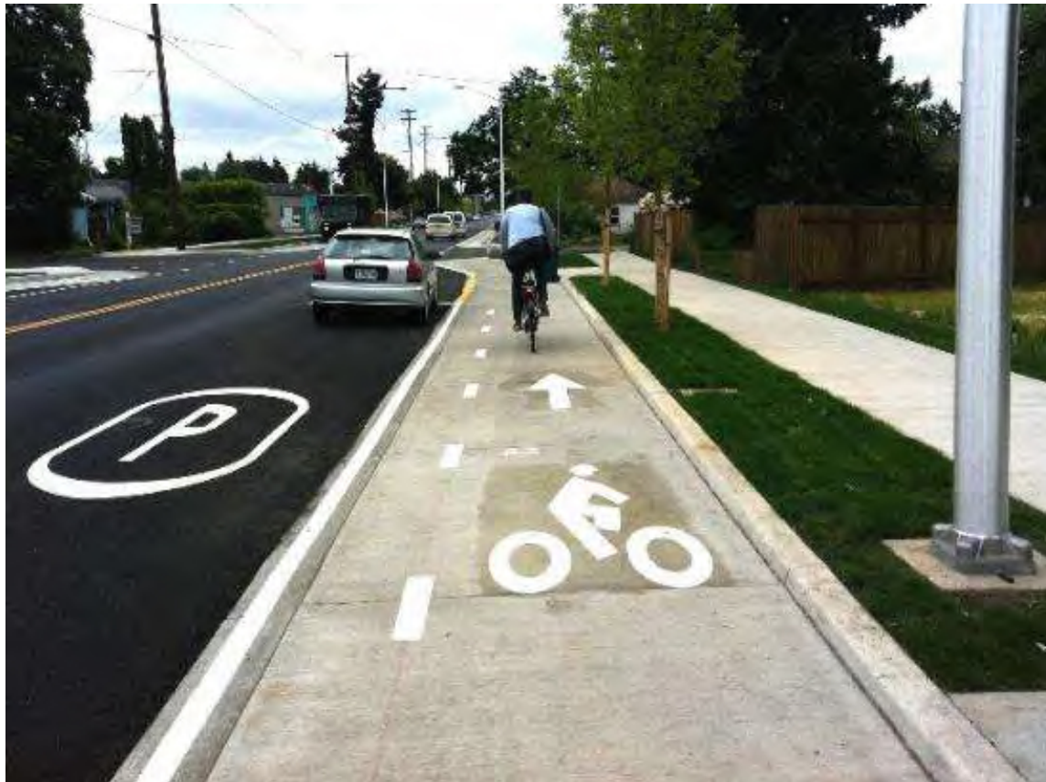
Example of a raised cycle track that is a Bicycle Parkway. Cully neighborhood, Portland. Photo: BTA
