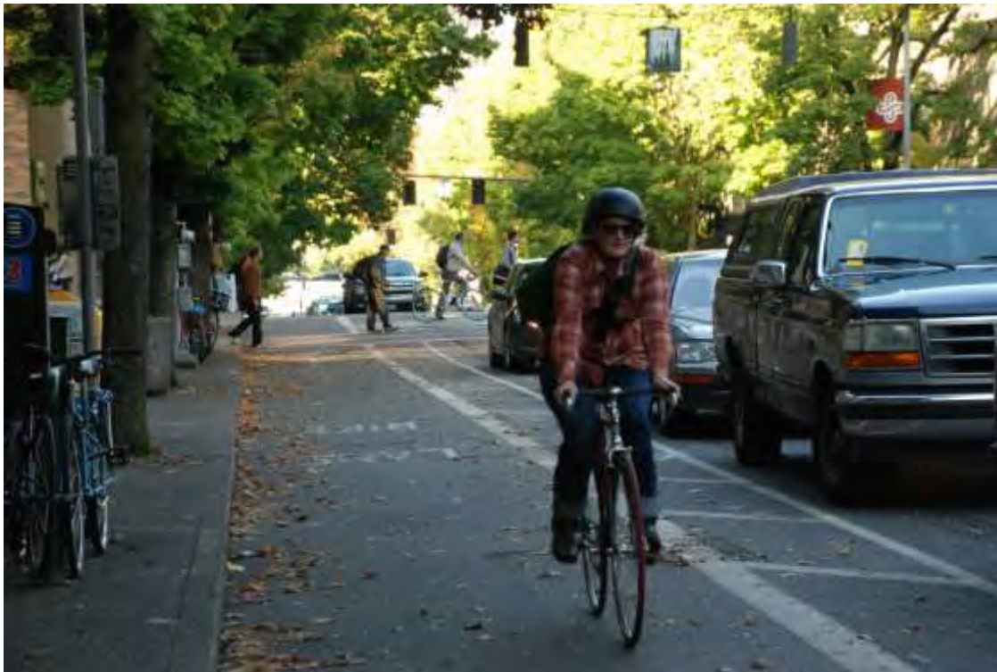
Providing separation for people walking and riding bicycles can make the road safer and easier to navigate for all users. Moving parked cars over provides a cycle track near Portland State University.
