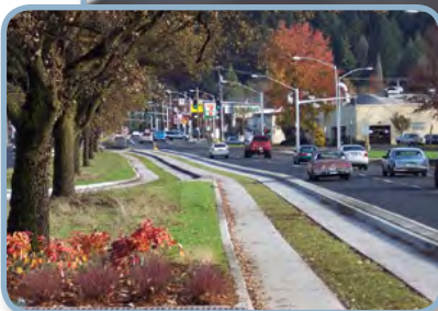
Eugene double track median guideway with landscaping
