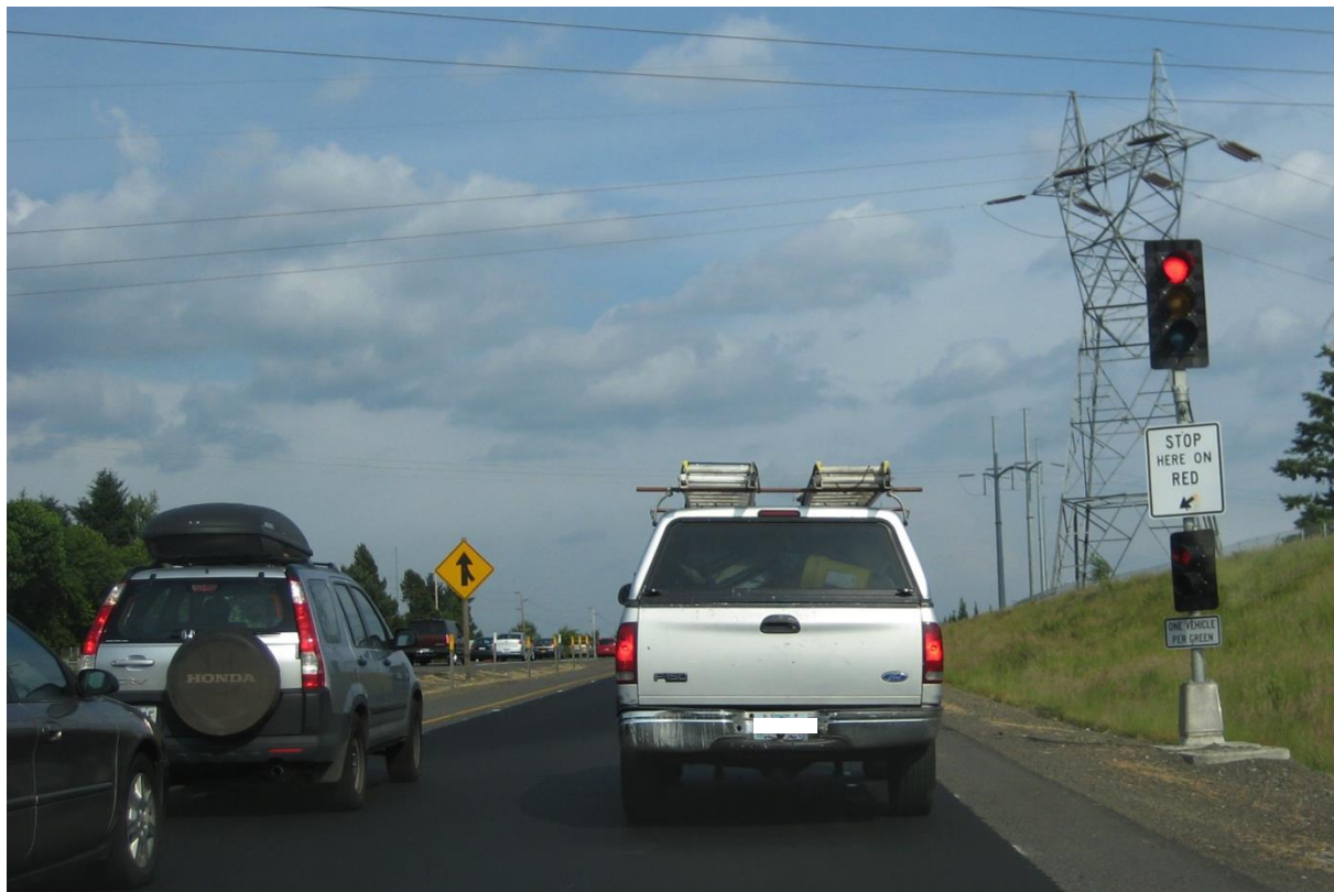
Figure 14: Ramp Meters Manage the Flow of Traffic onto Freeways
