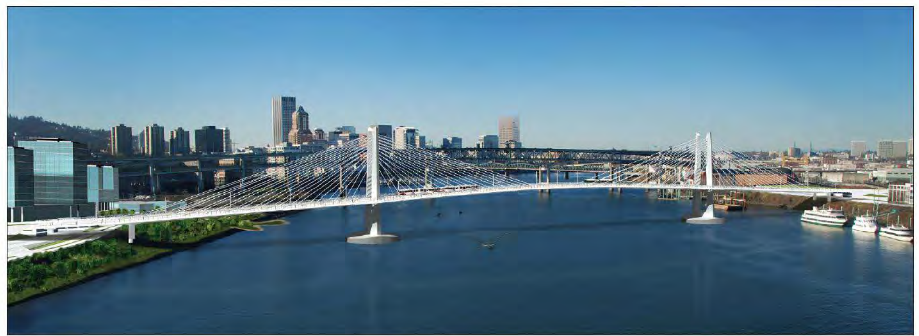
The Portland-Milwaukie Light Rail Bridge will carry light rail, buses, cyclists, pedestrians and eventually streetcars, but no private vehicles.
