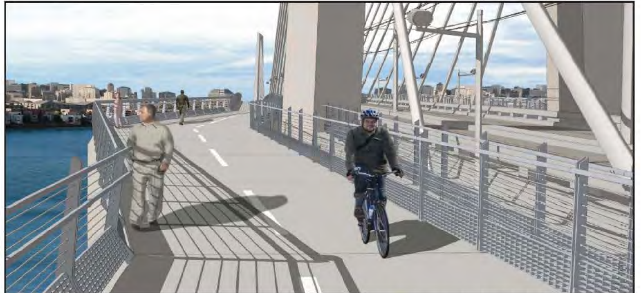
The Portland-Milwaukie Light Rail Bridge will have 14-foot bike-pedestrian paths on each side of the bridge, as well as extra width at the towers.
