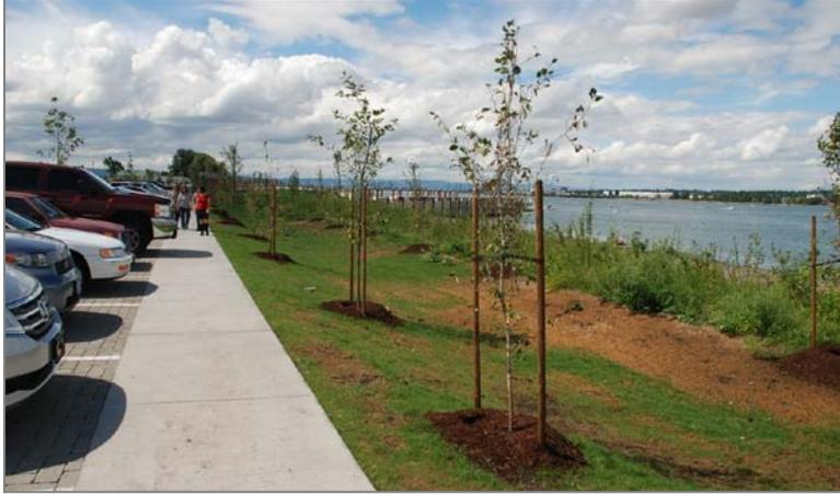
Expansion of Metro's **M. James Gleason Memorial Boat Ramp** on the Columbia River included the addition of over 117,000 square feet of native plantings, including infiltration bioswales that treat stormwater runoff from the parking lot, preventing it from entering the river, thereby improving water quality.
