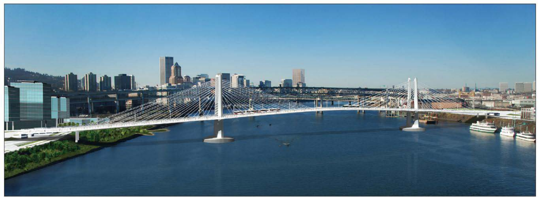
The Portland-Milwaukie Light Rail Bridge will carry light rail, buses, cyclists, pedestrians and eventually streetcars, but no private vehicles.
