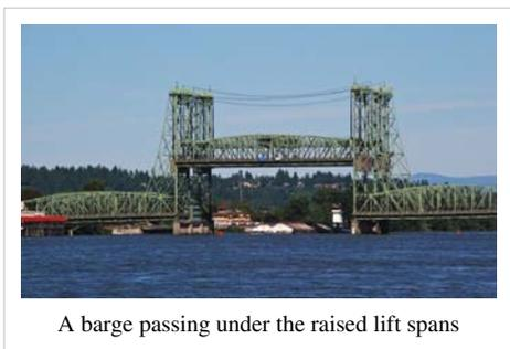
A barge passing under the raised lift spans
