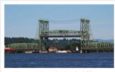
A barge passing under the raised lift spans
