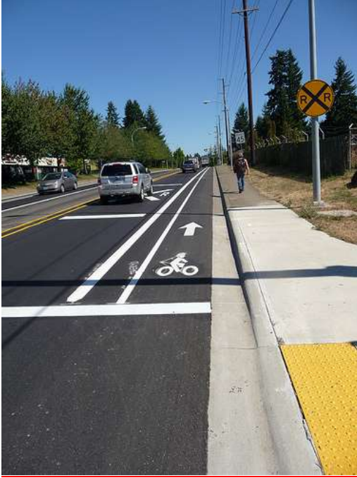
SW Tualatin-Sherwood Rd. buffered bike lanes (W. of Baler Way to Teton Ave; three-lane section) Regional Bikeway and Pedestrian Corridor
