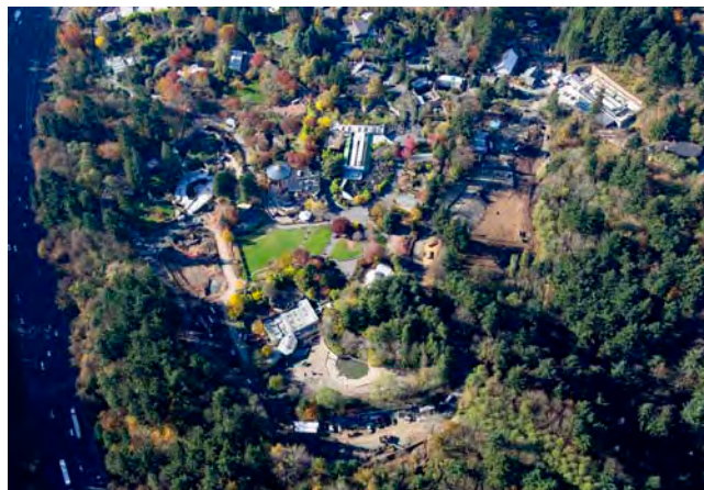
Zoo property aerial highlighting construction (Oct. 2013)
