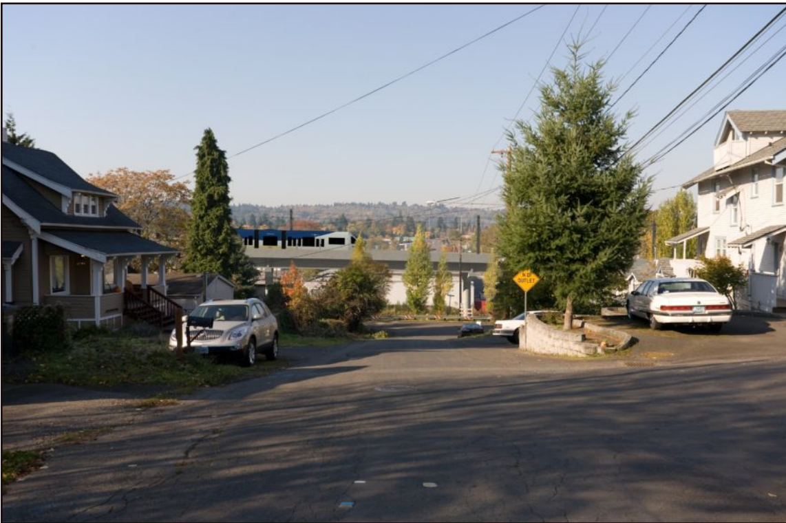
Figure D.8-1a Roswell Street: Tillamook Branch alignment View to the west
