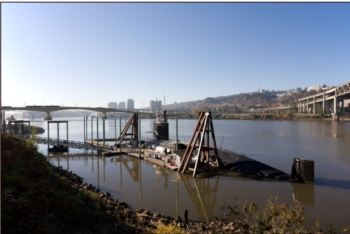
Figure D.4-1g Willamette River/OMSI: Porter-Caruthers - concrete segmental bridge View to the southwest
