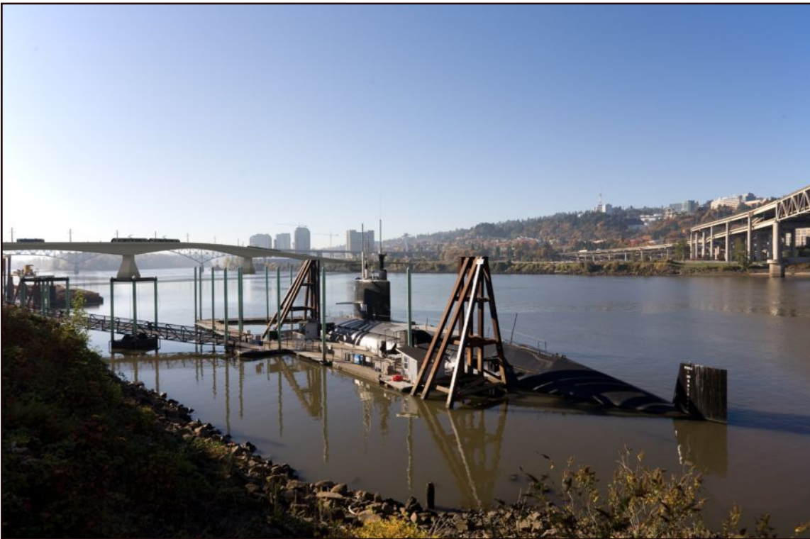
Figure D.4-1i Willamette River/OMSI : Porter-Sherman concrete segmental bridge View to the southwest
