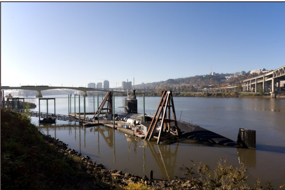
Figure D.4-1c Willamette River/OMSI: Meade-Caruthers - concrete segmental bridge View to the southwest
