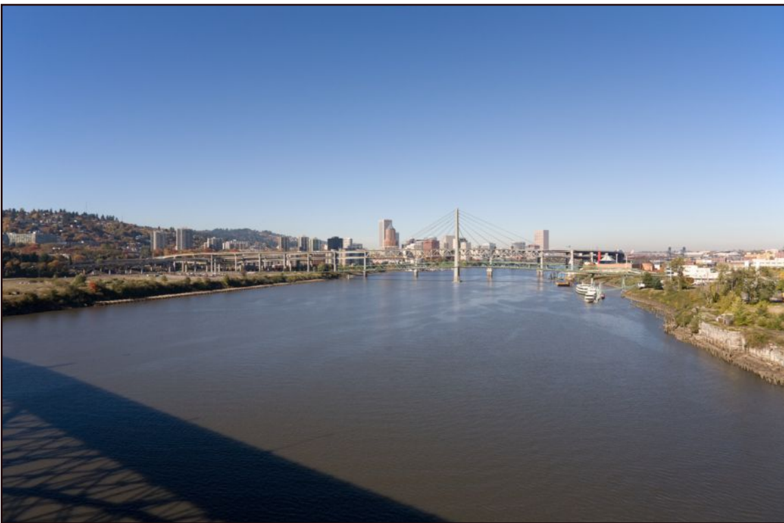
Figure D.5-1a Willamette River/Ross Island Bridge: 2003 Locally Preferred Alternative View to the north
