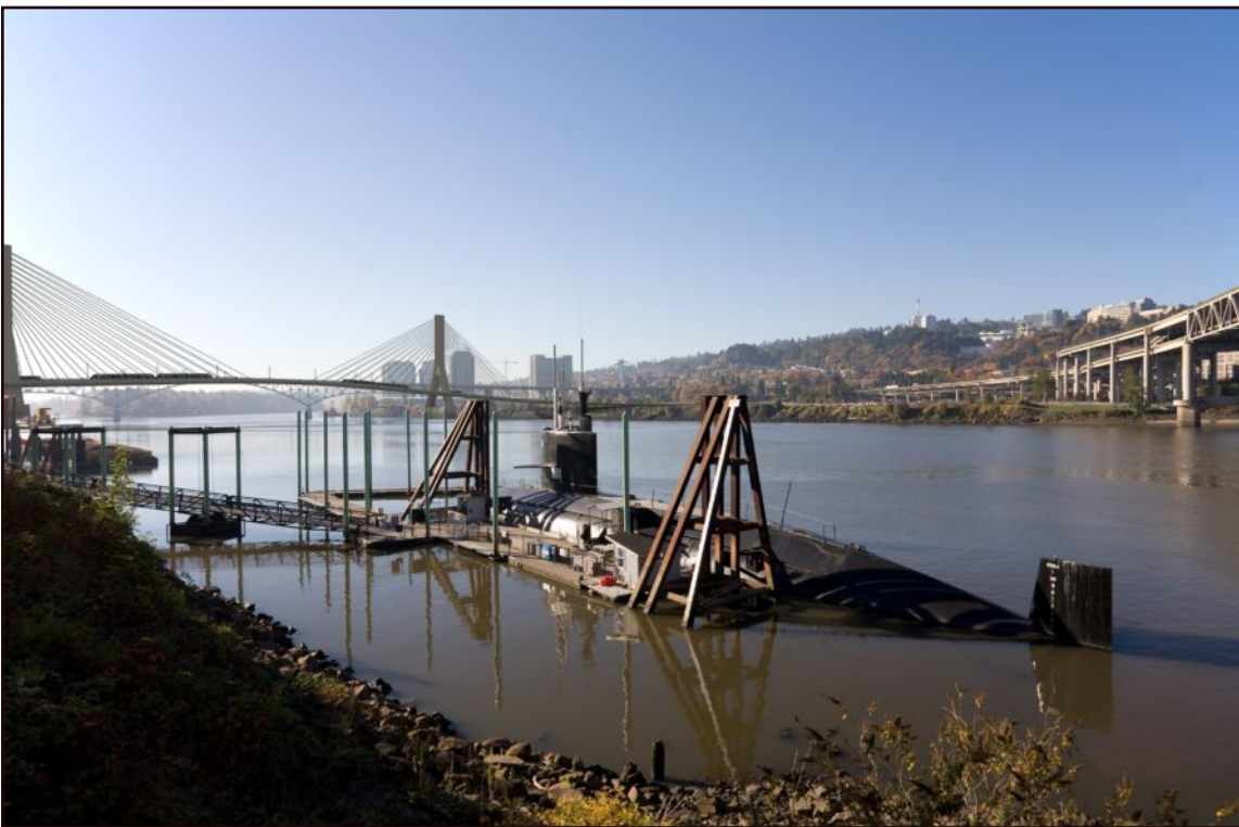
Figure D.4-1f Willamette River/OMSI: Porter-Caruthers - cable-stayed bridge View to the southwest
