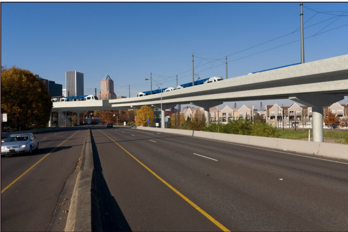
Figure D.3-1b Harbor Drive: connection to river crossing options in South Waterfront View to the north
