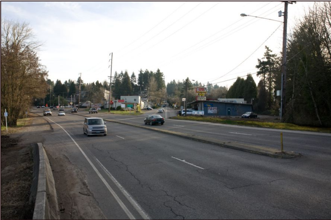
Figure D.15-1 Existing Condition - McLoughlin/Bluebird Street View to the south
