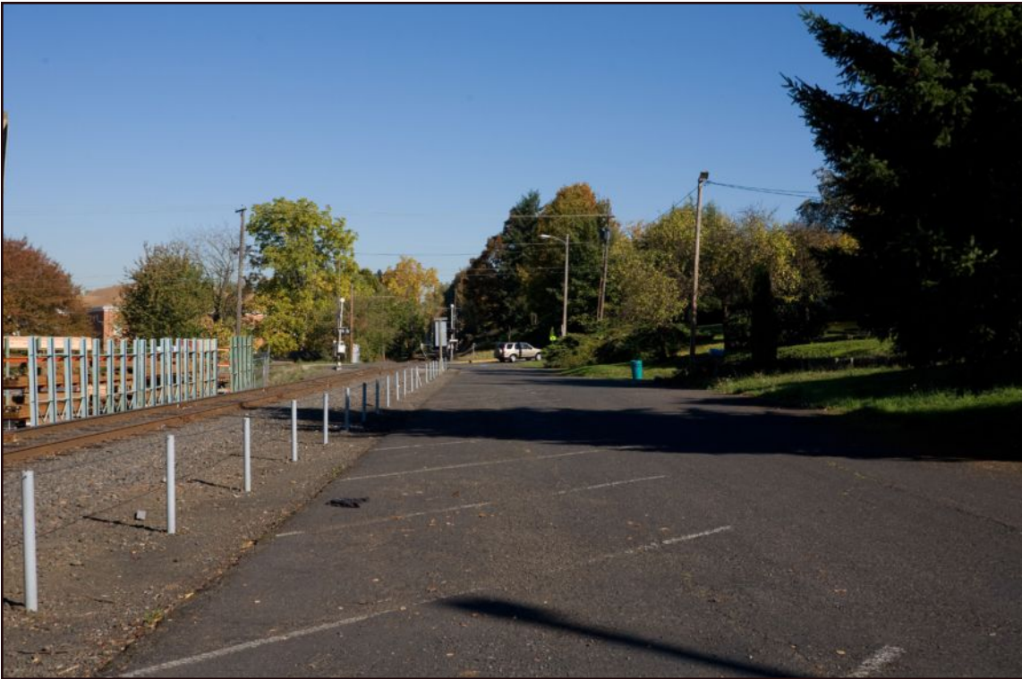
Figure D.10-1 Existing Condition - Monroe Street View to the north
