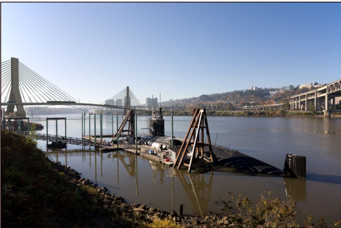
Figure D.4-1h Willamette River/OMSI: Porter-Sherman - cable-stayed bridge View to the southwest
