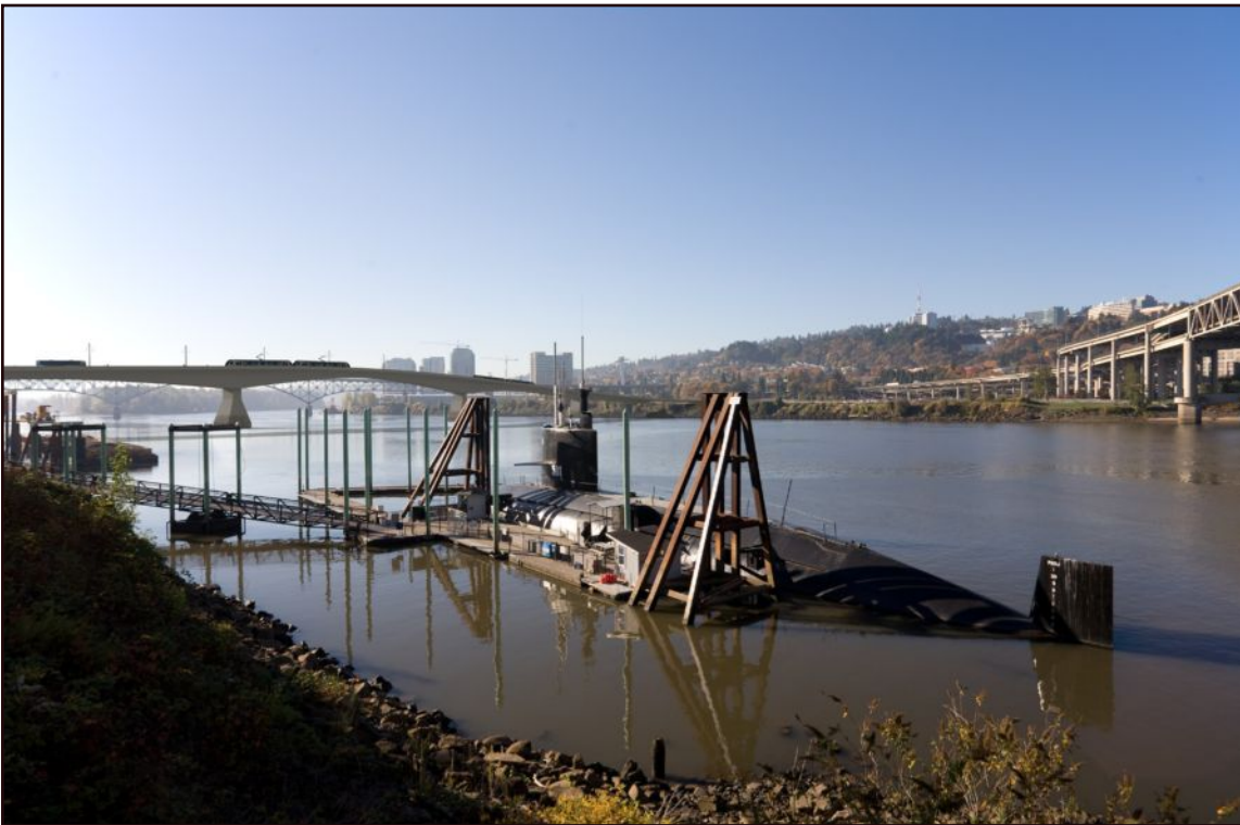
Figure D.4-1e Willamette River/OMSI: Meade-Sherman - concrete segmental bridge View to the southwest
