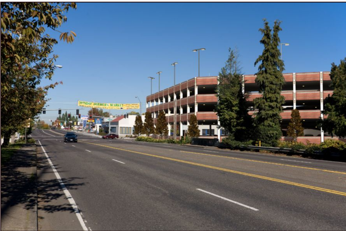
Figure D.12-1a McLoughlin/Lake Road: Lake Road Park and Ride View to the north
