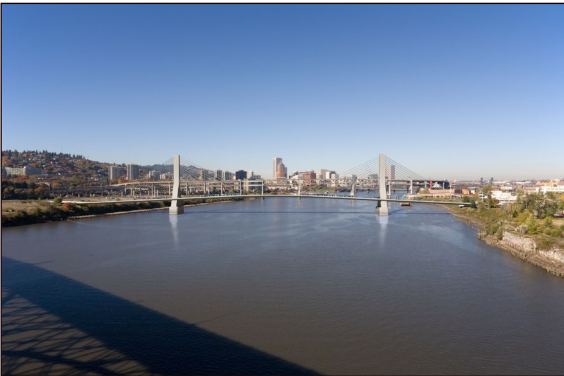
Figure D.5-1b Willamette River/Ross Island Bridge: Porter-Caruthers - cable-stayed bridge View to the north
