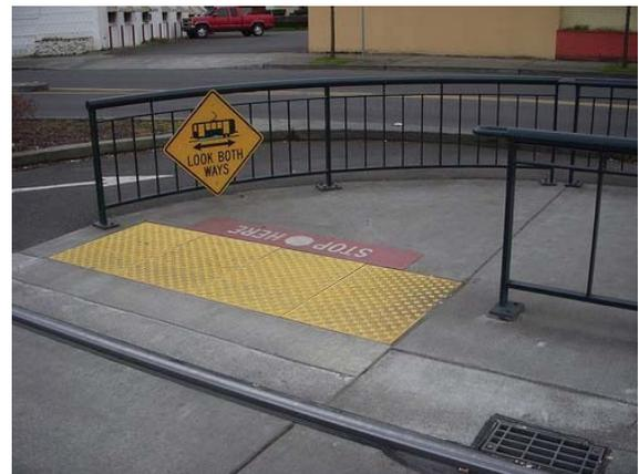
**Figure 9. Bike route crossing MAX tracks on Interstate at off-set intersection**
