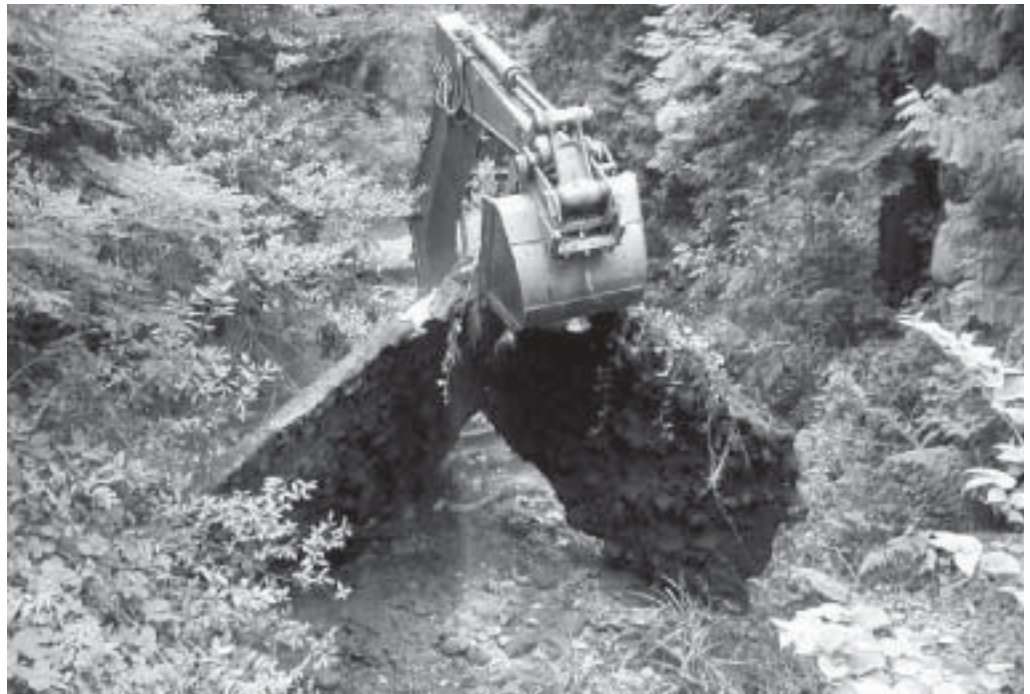
In August 2001, Metro removed a dam from Johnson Creek on its Ambleside open space property in Gresham to improve fish passage.
